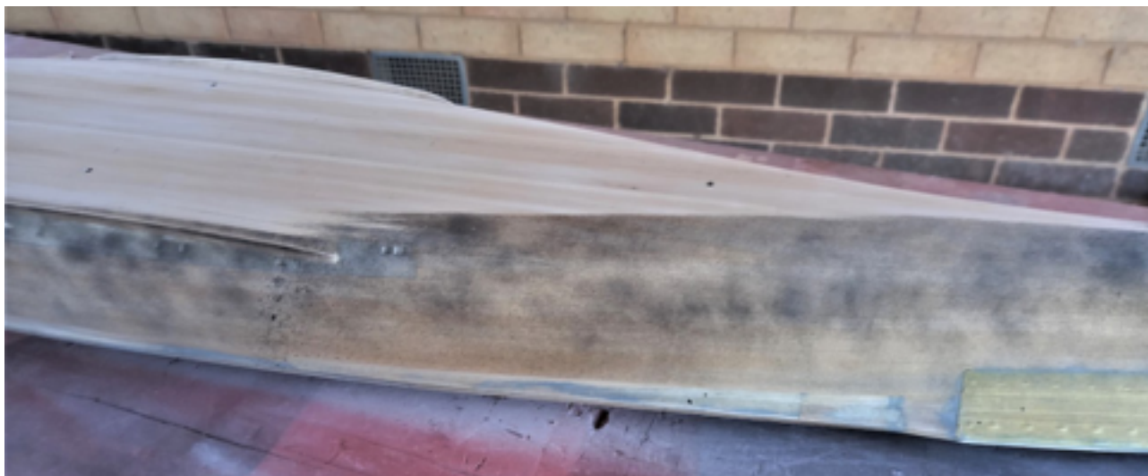
Dusting of black paint, bottom already sanded.
