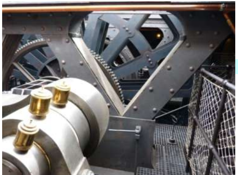
A small section of the massive steam plant.
