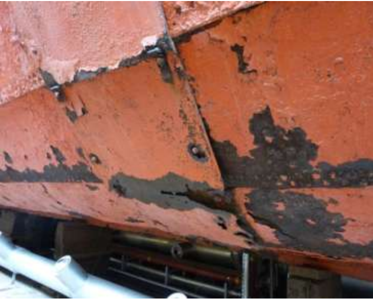
The hull below the water line is in fairly poor shape due to its years of neglect in the Falklands.
