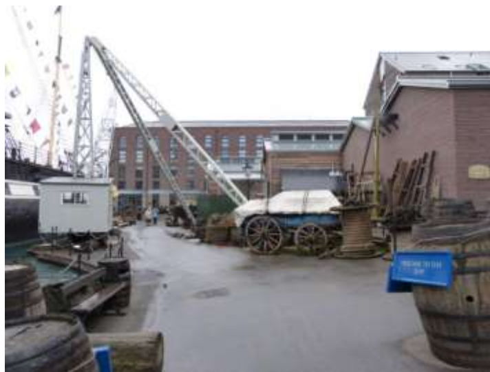
Another view of the wharf area. Note the crane, further along the river towards the city is an original working steam crane, also worth a visit for steam enthusiasts.
